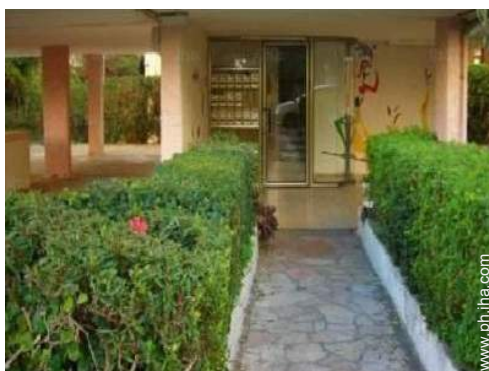
Restored apartment house/building
