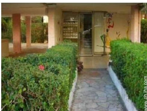
Restored apartment house/building
